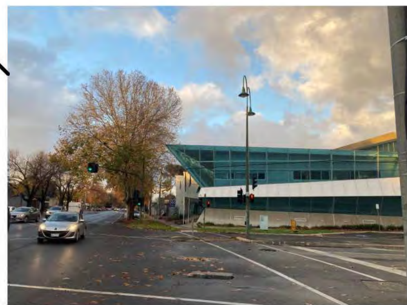
Bendigo Police Station 3 Stores
