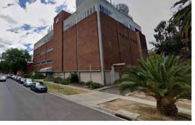
Communications Building 4 Stores
