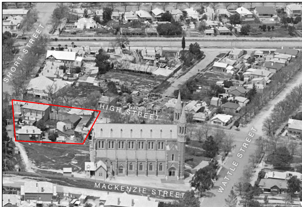
Figure 3 Annotated c.1934 oblique aerial view south, showing the Cathedral as still only partially completed. The approximate development area is indicated in red, and it is noted that all of the buildings visible at this time have since been demolished. Source: State Library.
