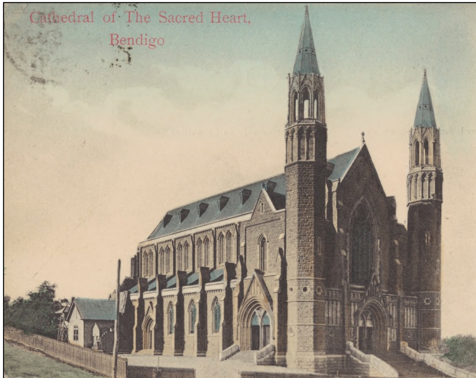
Figure 2 c.1904 view of the Sacred Heart Church from the west after the completion of the nave, aisle and western lantern towers, and before the construction of the main tower, spire, and chancel. Source: State Library Victoria.
