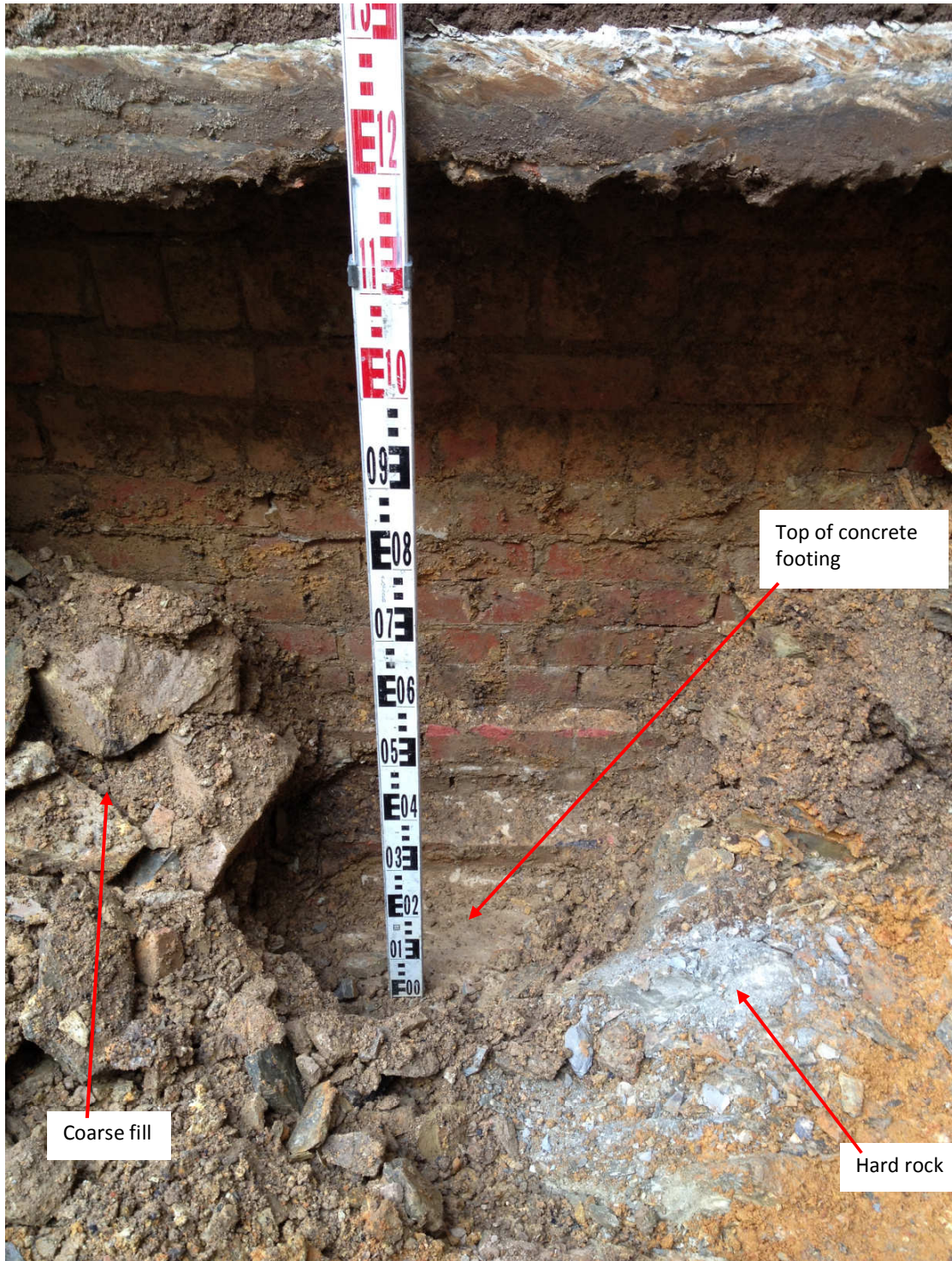
Fig 1: Footing Exposure
