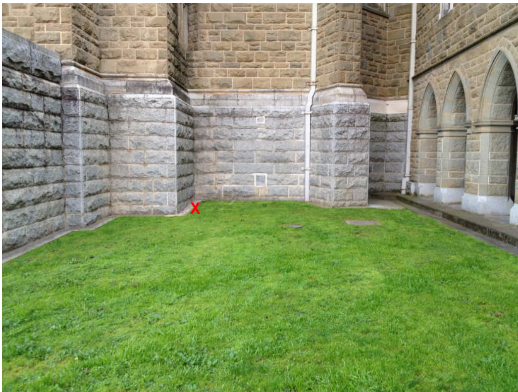
Fig 3: Location of footing exposure
