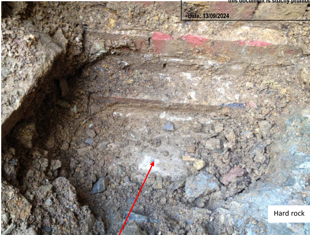
Fig 2: Top of concrete footing (closer view)
